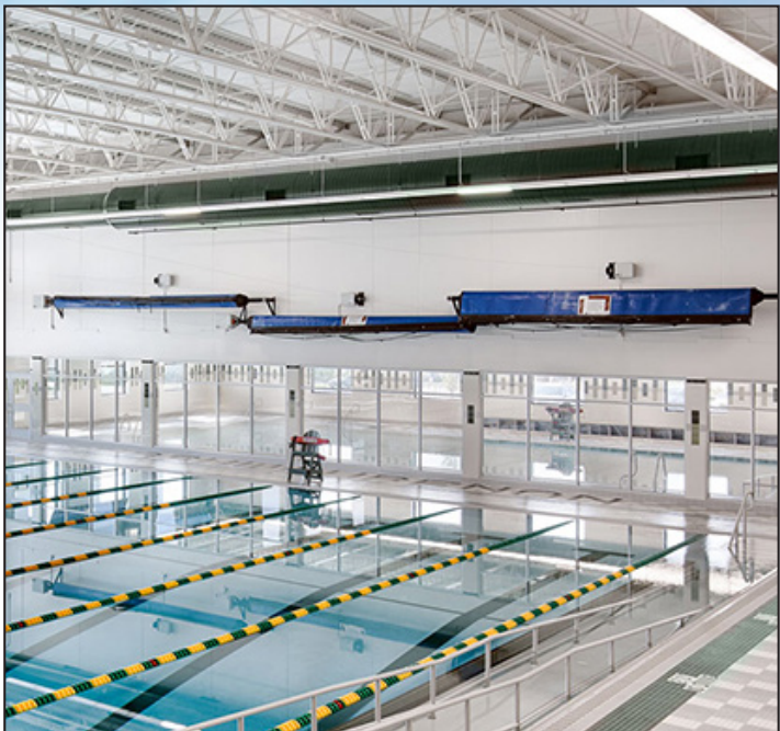
No lost deck space
